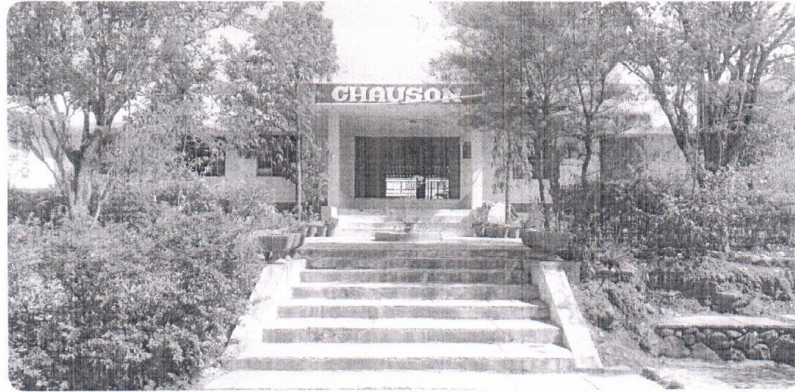
Front view of the Building
