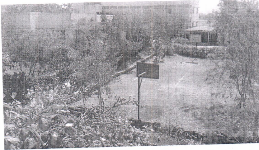
Rear view of the building
